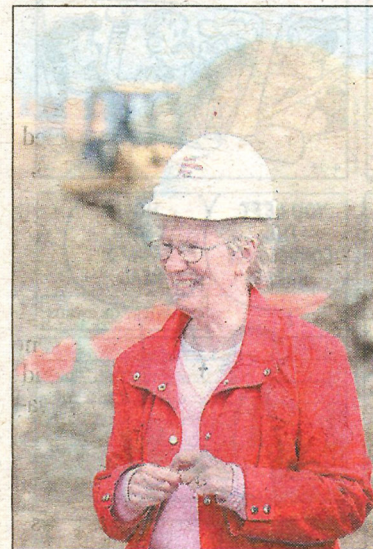
Sister Rose Helene Wildenhaus, vice president of the St. Mary Development Corp., supervises the Lyons Place construction site, a 67-unit senior housing facility in east Dayton. Staff photos by Chris Stewart
